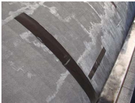
After 71 years the roof covering has given way to the elements and is in need of replacement.
