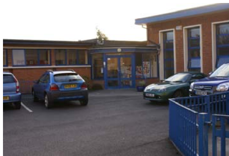
The Primary School is on a tight site!
