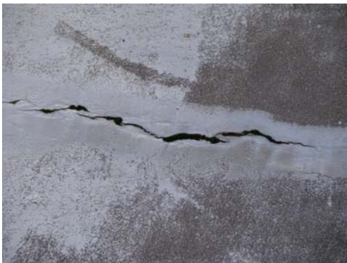
After 71 years the roof covering has given way to the elements and is in need of replacement.
